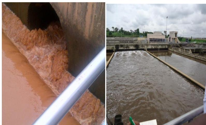
Wastewater inlet chamber and bioreactor at Wupa water treatment plant Abuja
